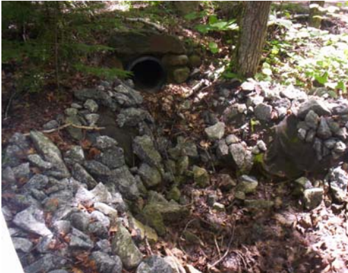
Plunge pool and outlet protection
