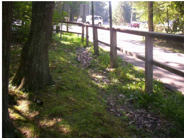
Grassed waterway to dissipate stormwater volume, reduce erosion and stop harmful pollutants and nutrients from entering the surface water.
