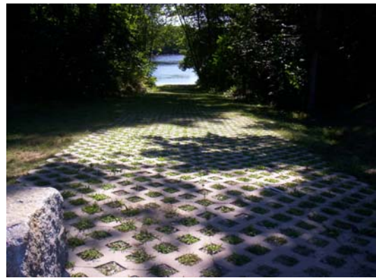
Pervious paver boat ramp
