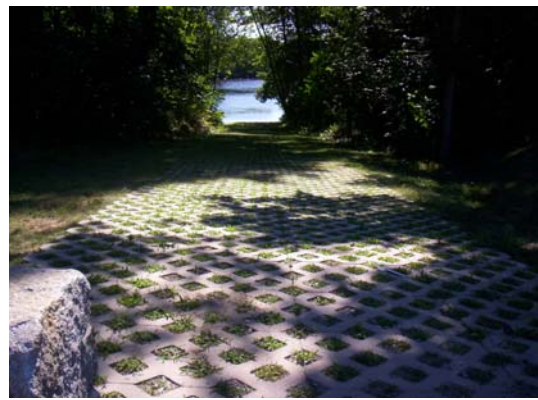
Pervious paver boat ramp
