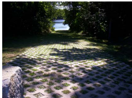
Pervious paver boat ramp
