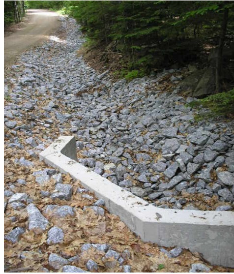
Stone lined apron and rock rip rap
