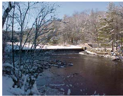
West Henniker Dam, rebuilt in 1936 on the site of dams dating back to the 1700s.
