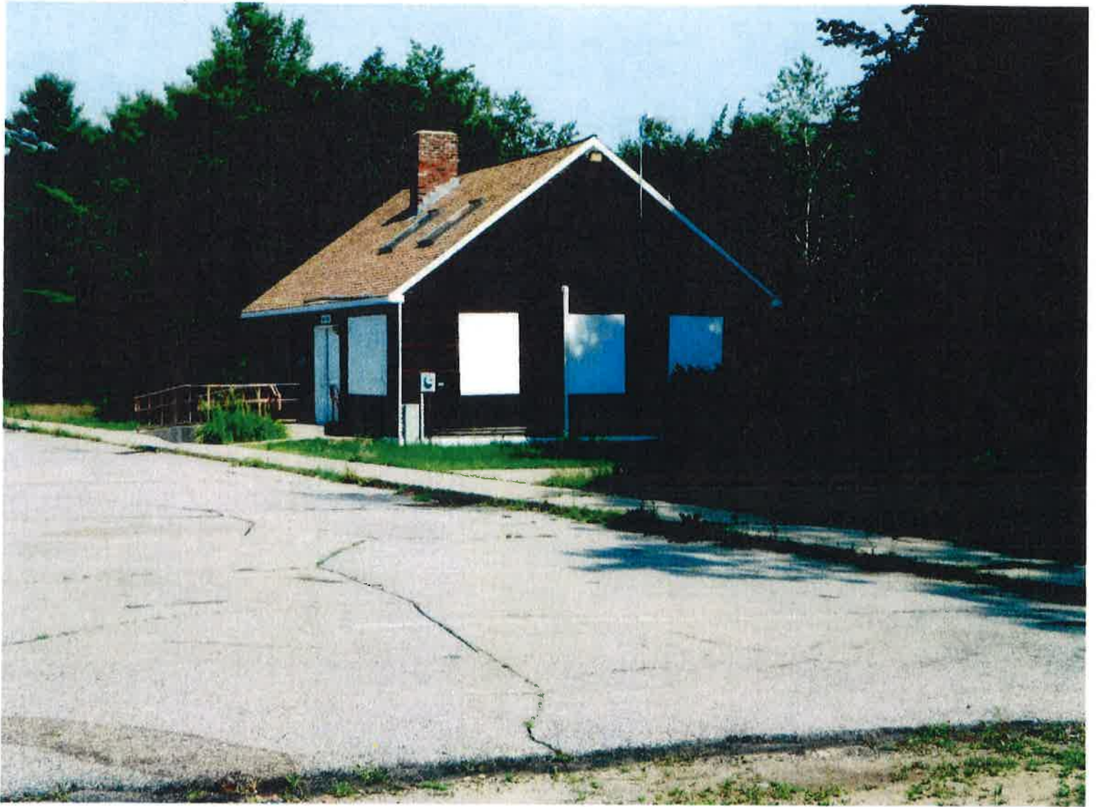
Rumney Rest Area
