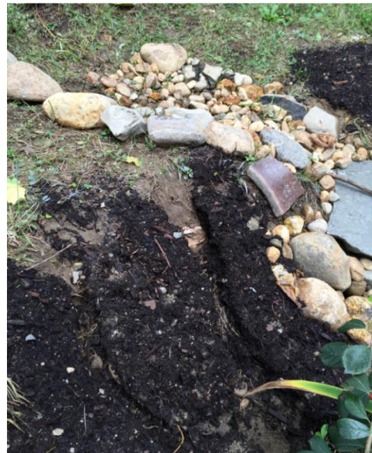
This rain garden inlet required an adjustment after the first large storm. Stone was added to capture runoff from a wider area.
