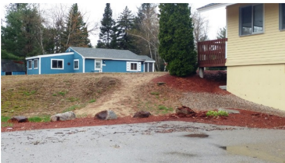
Eroded pathway from side area to back parking lot Date: 5/2/17
