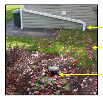
The downspout extension was placed in a trench underground and connected to the inlet pipe
