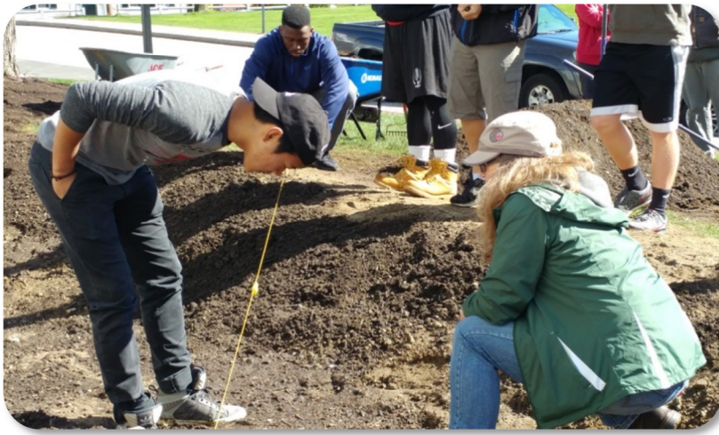
PEA students use a line level and shovel lots of soil while learning to build a rain garden.
