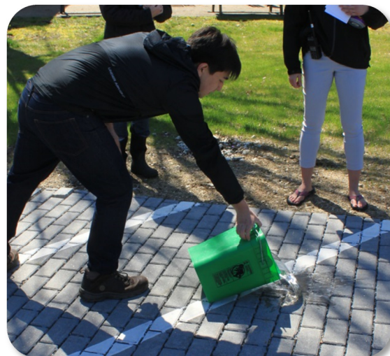
Porous pavers behind the Lamont Health & Wellness Center allow rain and melting snow to pass through to an infiltration basin below.
