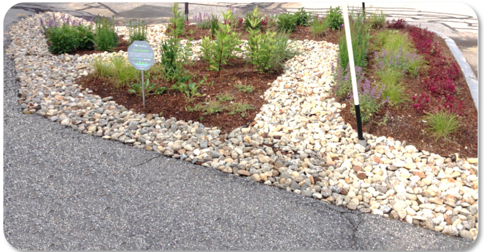
NHTI repurposed a raised traffic island to create a rain garden which captures stormwater outside the Goldie Crocker Wellness Center.
