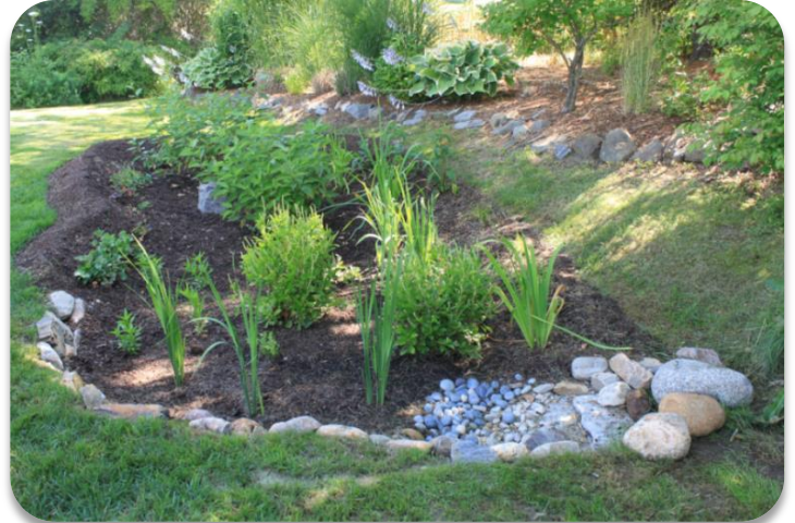
The finished rain garden with the reinforced inlet shown in the foreground.
