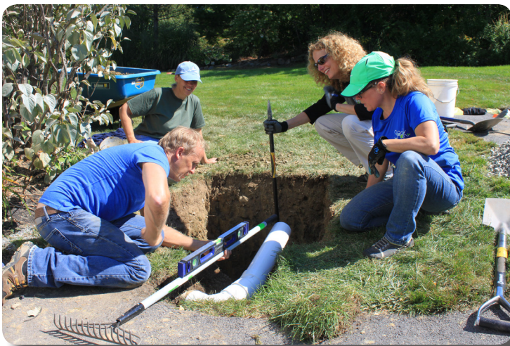
An overflow pipe is installed to drain excess flow during larger storms. Geotextile fabric prevents soil and sediment from migrating into the dry well.
