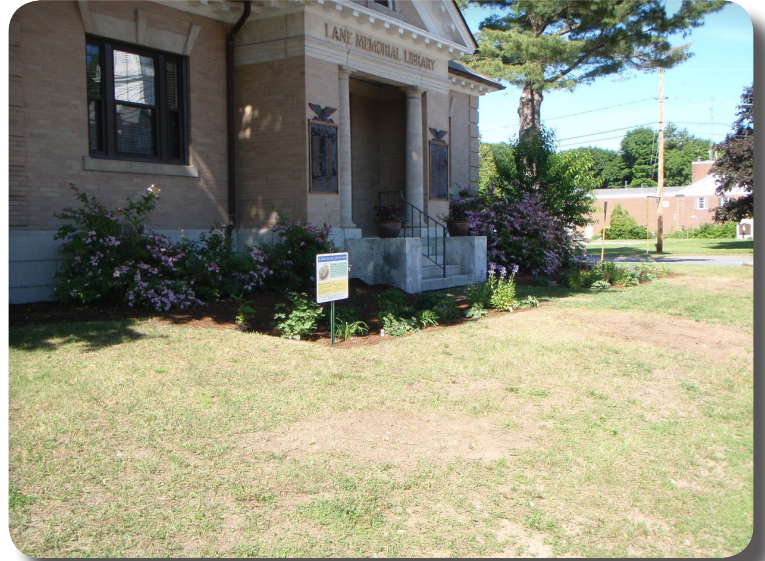
The finished rain garden receives runoff from the roof of the Lane Memorial Library
