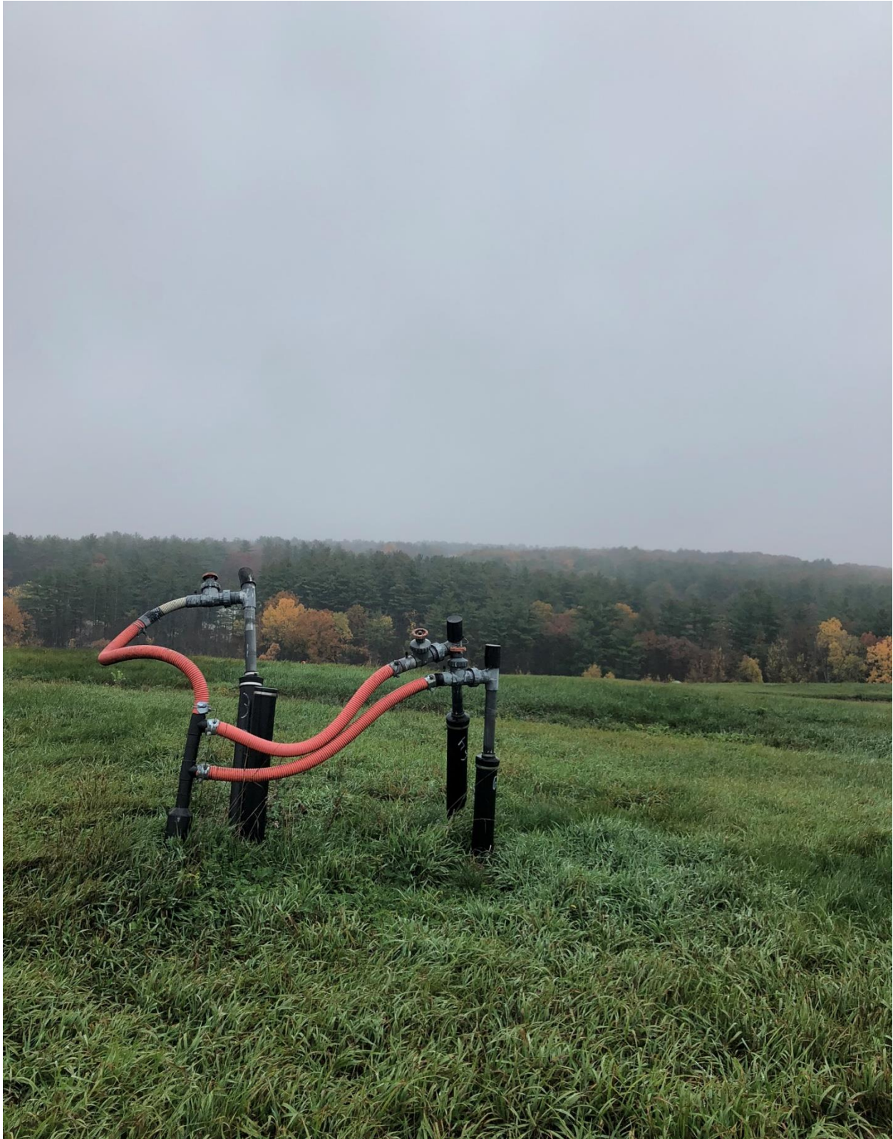
5. View of landfill gas collection wells and over top of capped landfill looking to the north.
