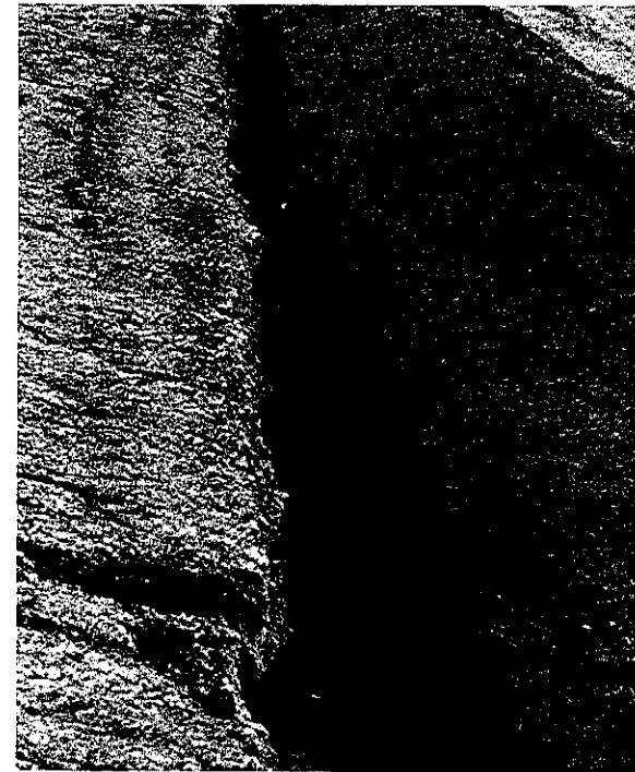
Fig. 7.28 Eroding swale/dike; lining is needed.
