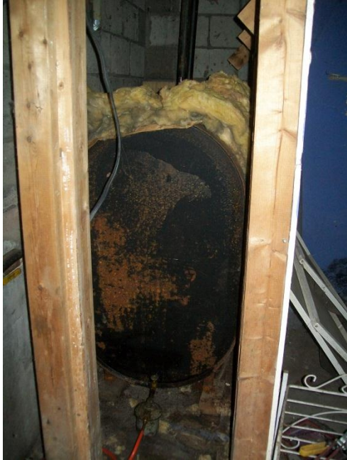
View of the 275-gallon fuel oil AST in basement of #4 Oak Street Extension.
