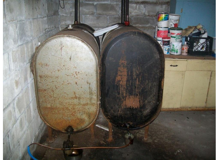
View of two fuel oil ASTs located in the basement of #22 Oak Street Extension. Note: slight petroleum staining on the floor likely from a surficial spill during a filter change.
