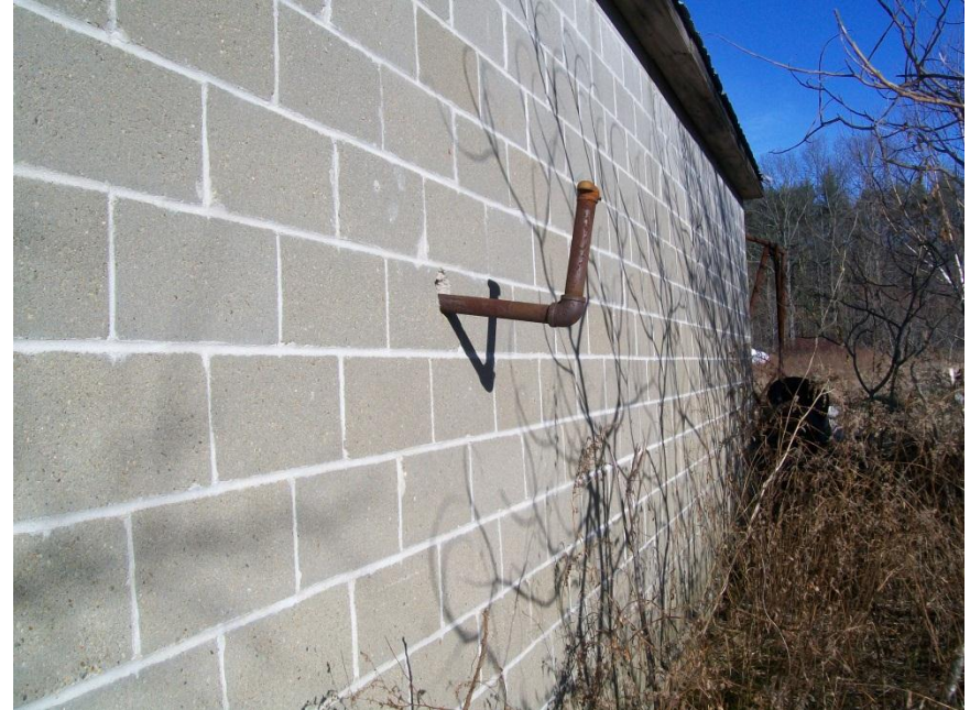
View of a potential AST vent pipe protruding through the rear wall of the three bay garage looking northeast.
