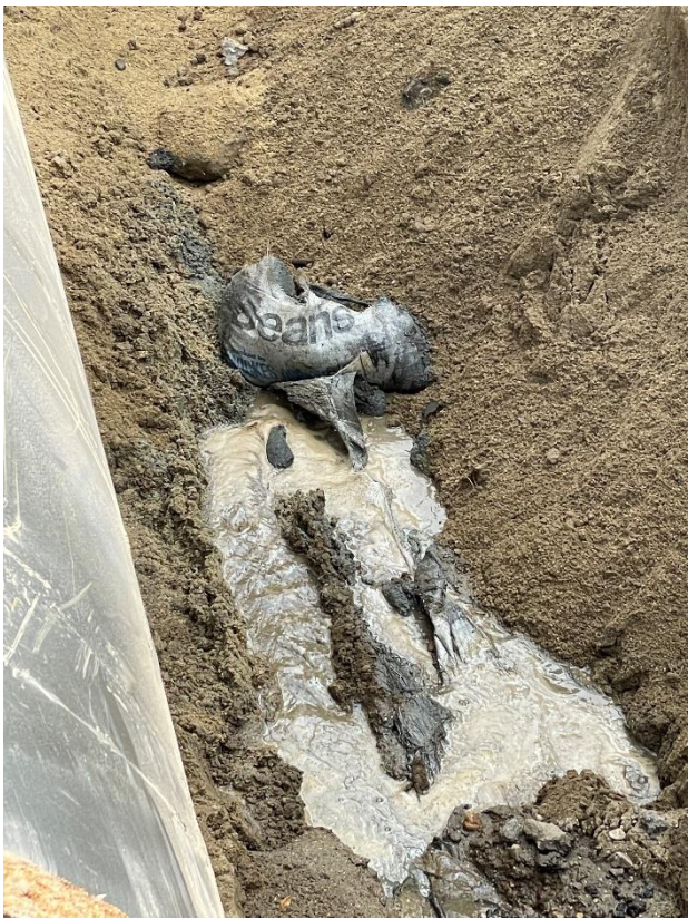
Photos 5 & 6: Accumulated groundwater at base of Tank No. 6 excavation, product sheen observed on groundwater surface.
