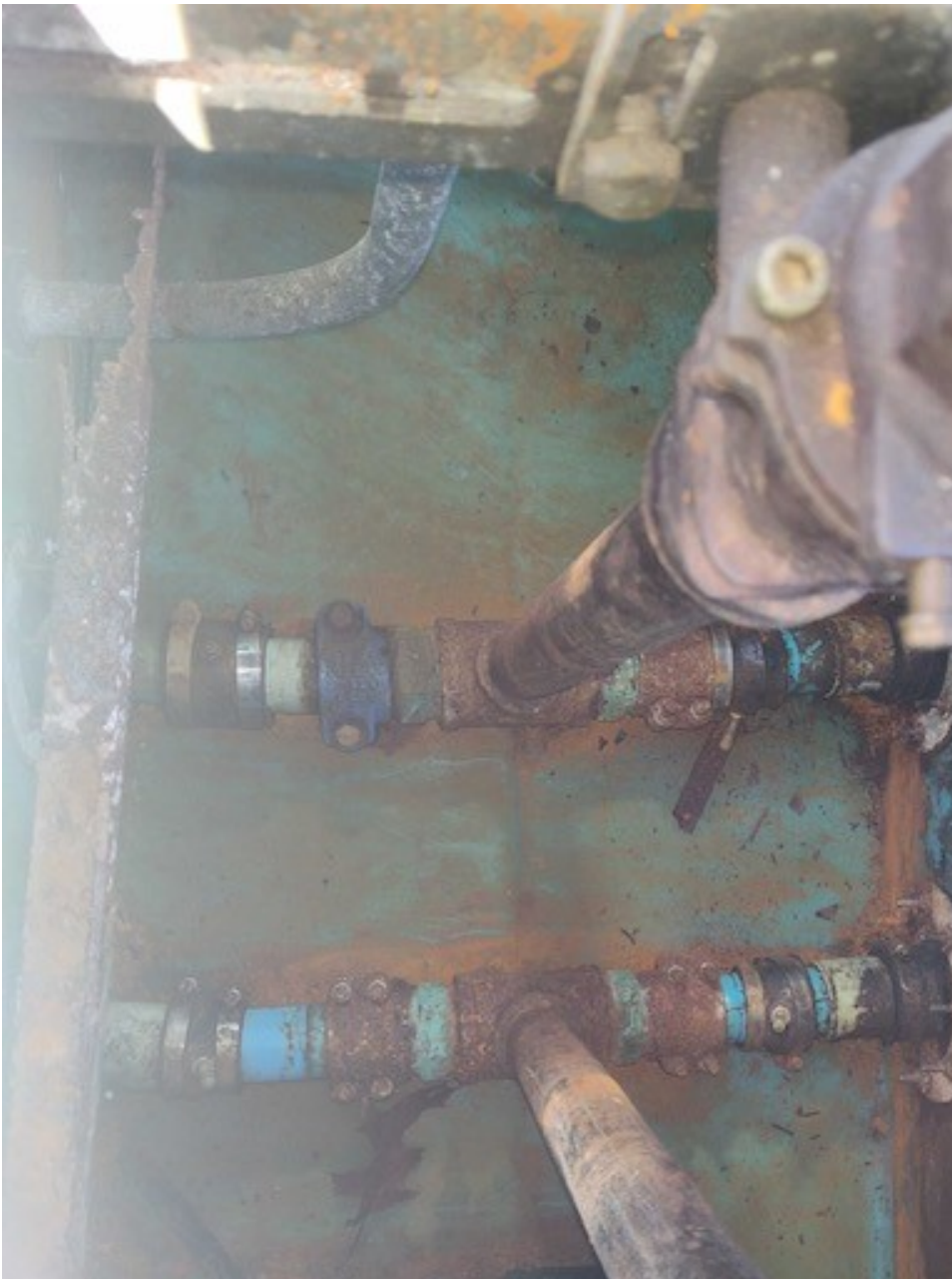
primary has a slit down the middle on the top part of the primary line inside dispenser.
