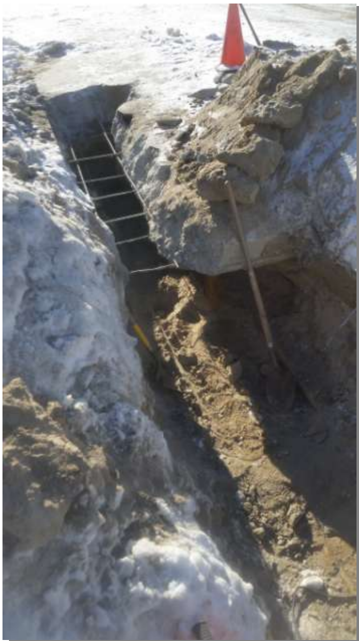
PHOTO #4 PIPING ALONG TOP OF UST
