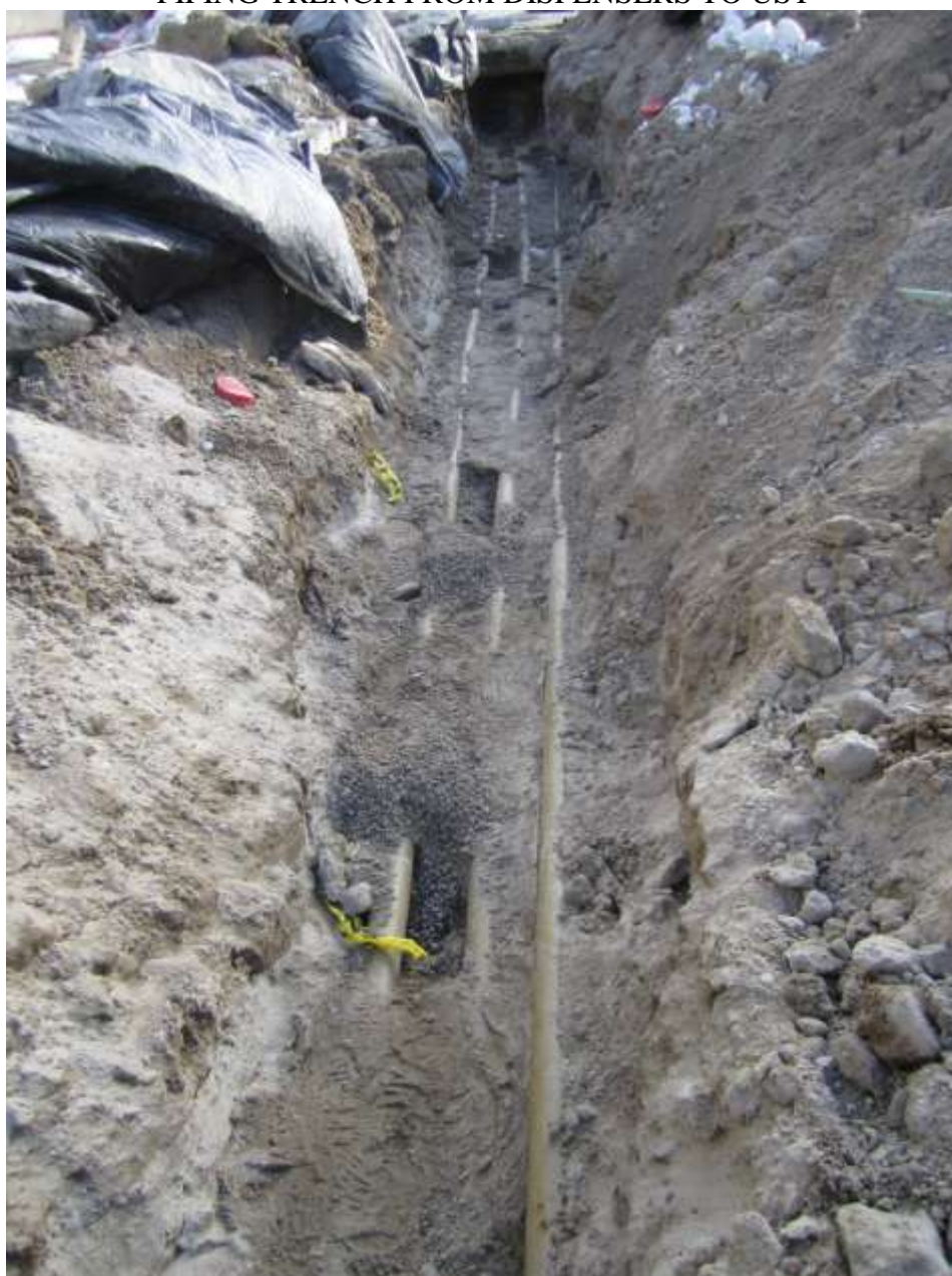
PHOTO #2 PIPING TRENCH FROM DISPENSERS TO UST
