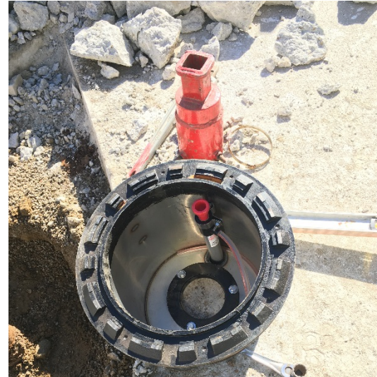
Photo 2: (10/17/2017) View of new spill bucket.
