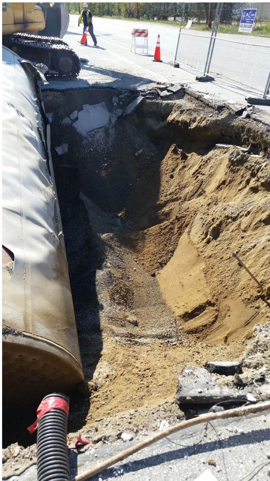
3. UST grave following the removal of the 3,000-gallon tank.
