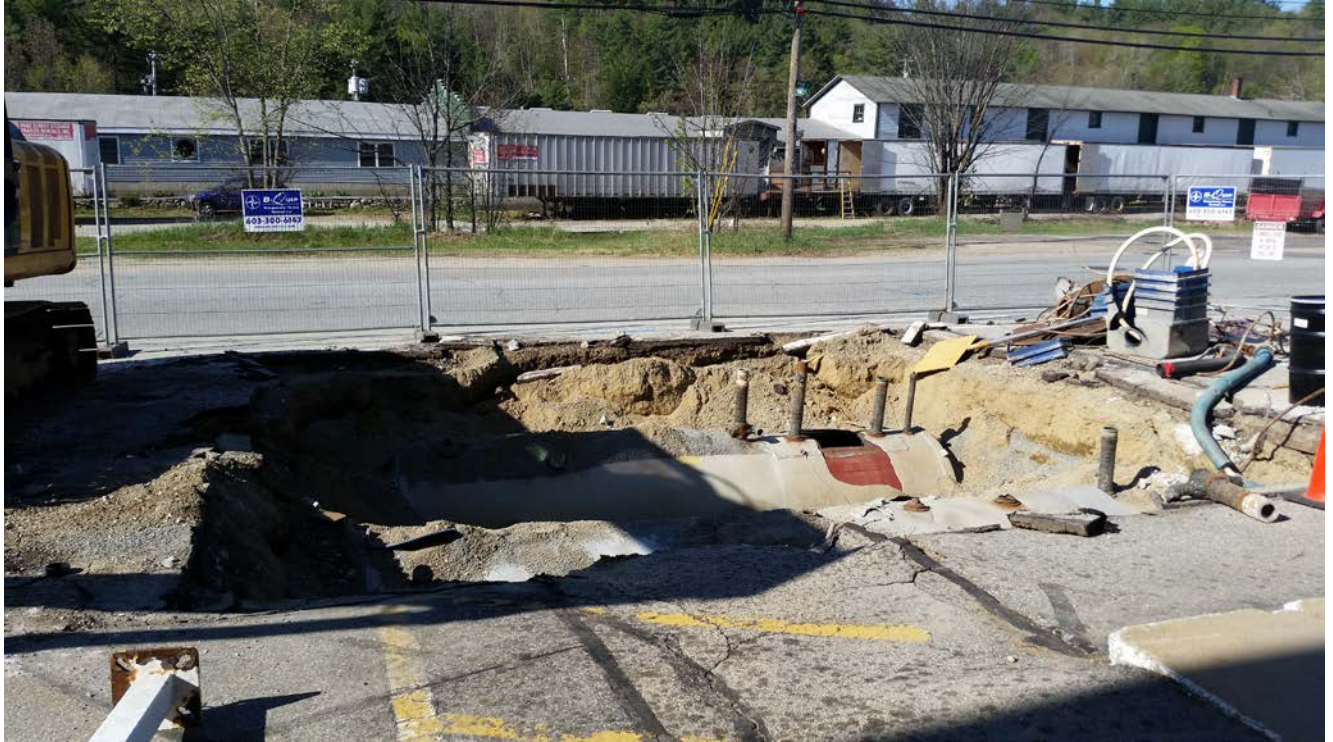
1. Top of gasoline USTs following pad removal, venting, cutting, and cleaning (view is to the south west).
