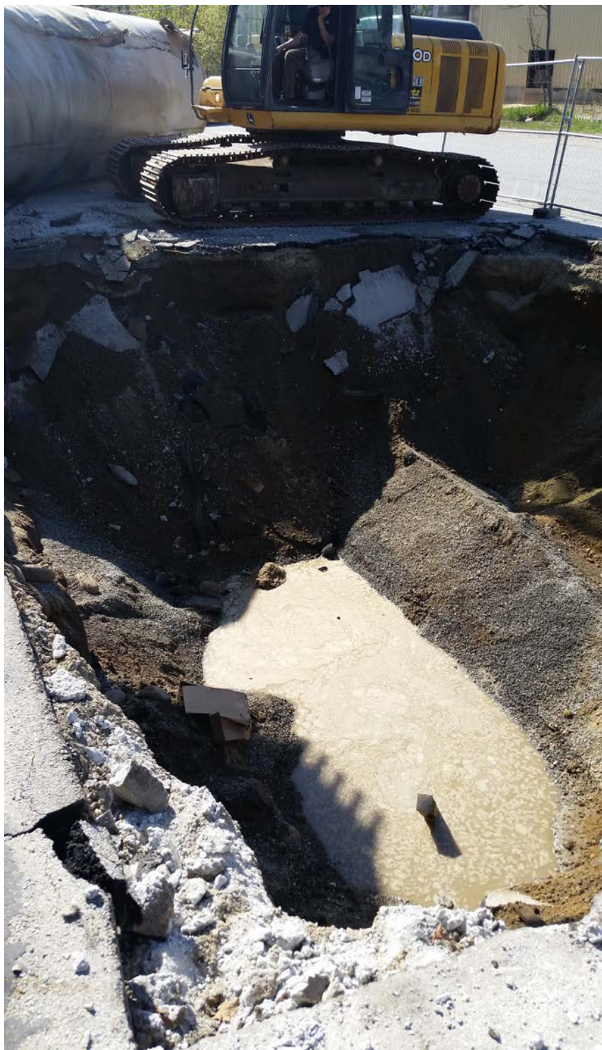
6. Groundwater encountered below the 8,000-gallon UST at approximately 10 feet below ground surface.
