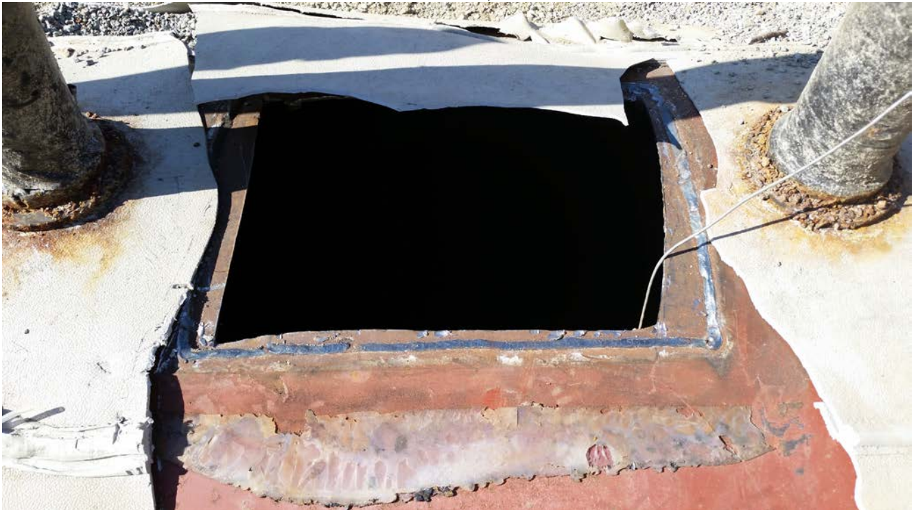
2. Gasoline UST entry point; note previous welded patch (typical of two).
