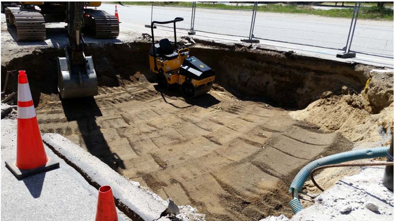
8. Backfilling and compacting following UST(s) removal.
