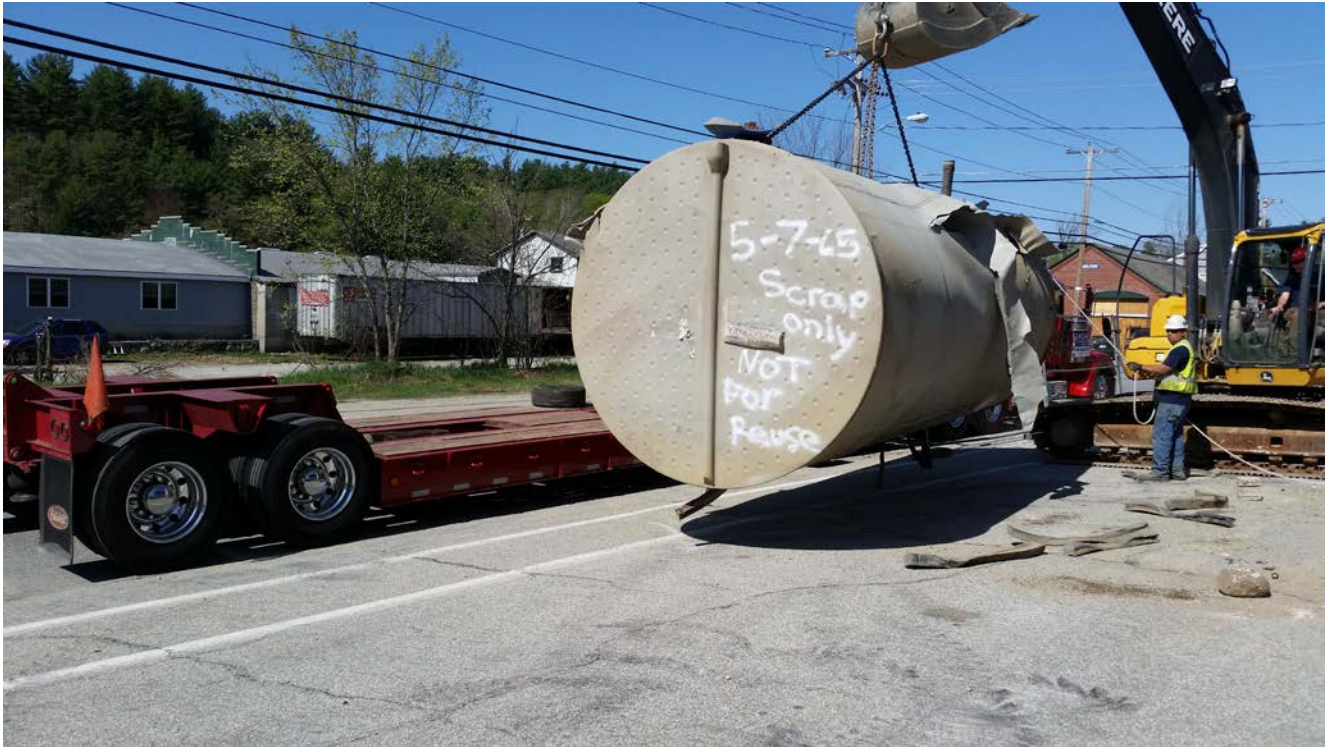
7. UST being loaded for offsite scrap disposal (typical of two).
