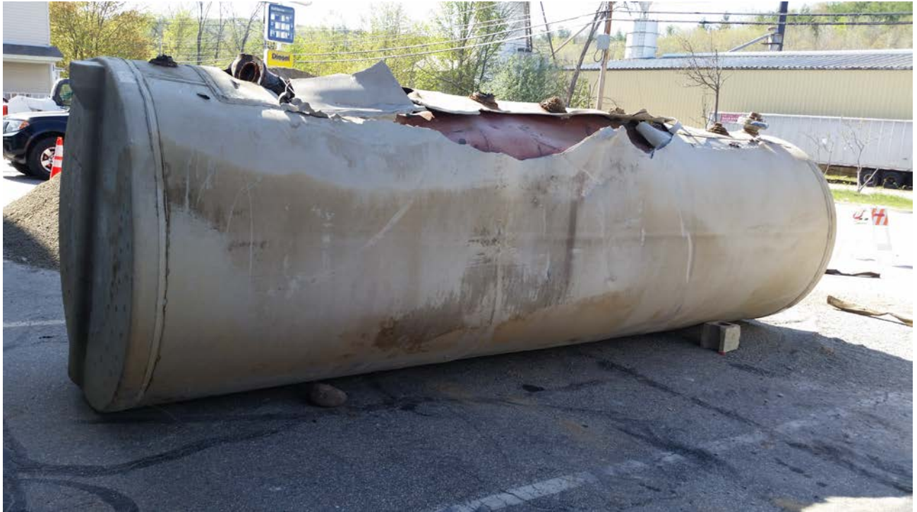
4. 3,000- gallon Gasoline UST following removal; no rips, holes or tears were noted (note plastic welded containment around tank).
